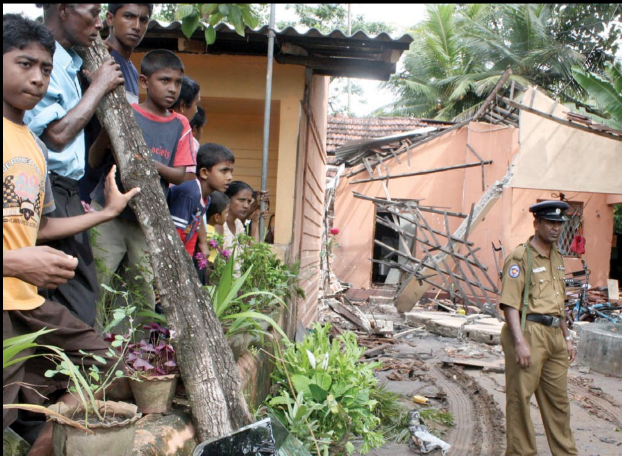
The front portion of the family home was reduced to rubble
